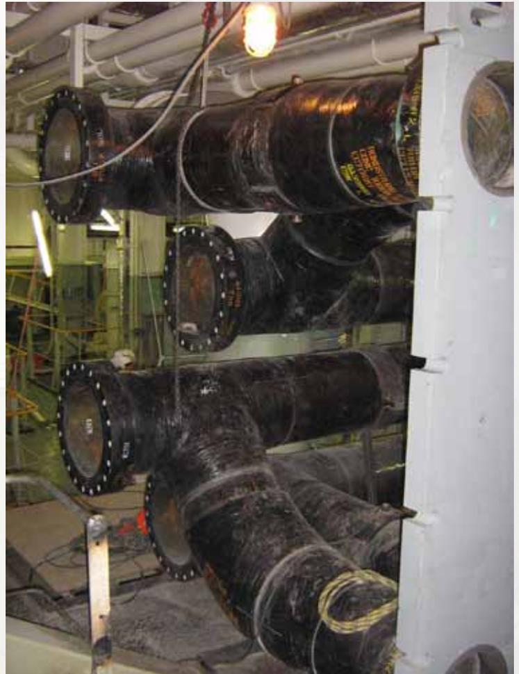
*Bondstrand connection to front plate box cooler*
