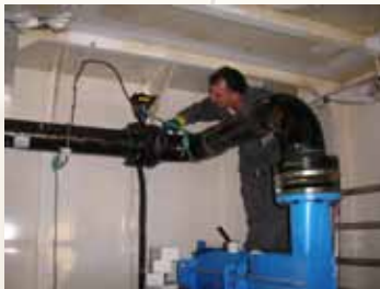
Pipe installation in engine room
