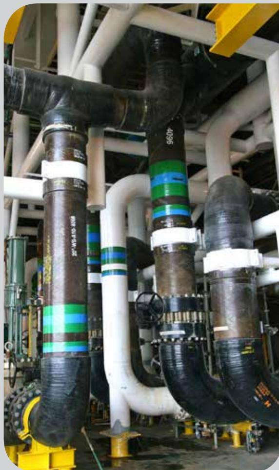
The question to ask is, Do you have to accept repeated pipe replacement due to corrosion problems in your seawater piping? The answer is: No. Corrosion problems can be eliminated with BONDSTRAND™.
