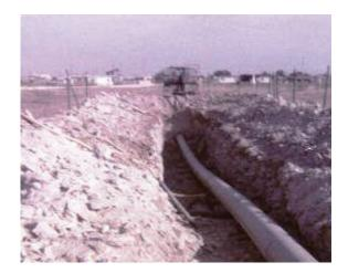
Application: Steel reinforced concrete pipe carrying brackish water was rupturing due to corrosion and water hammer.
